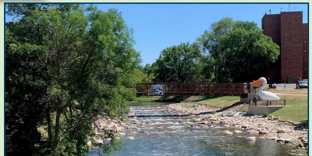
The deteriorating dam in Pelican Rapids, MN was modified into a Rock Arch Rapids winter 2022/2023. The ramp gradually steps down the water 5 feet over 12 arches.
